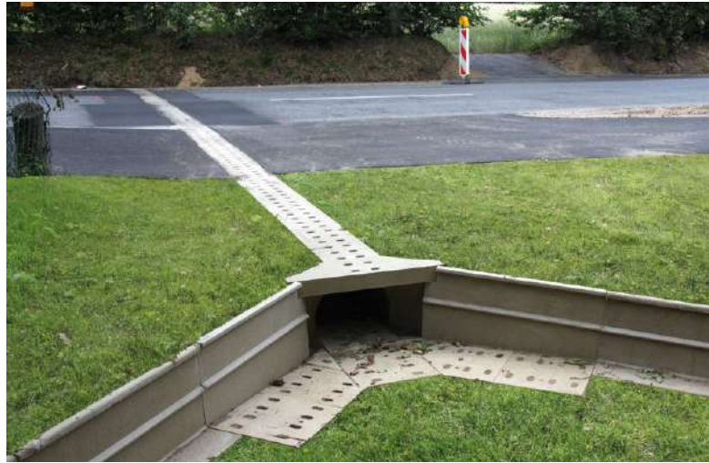
KT500 fauna tunnel
