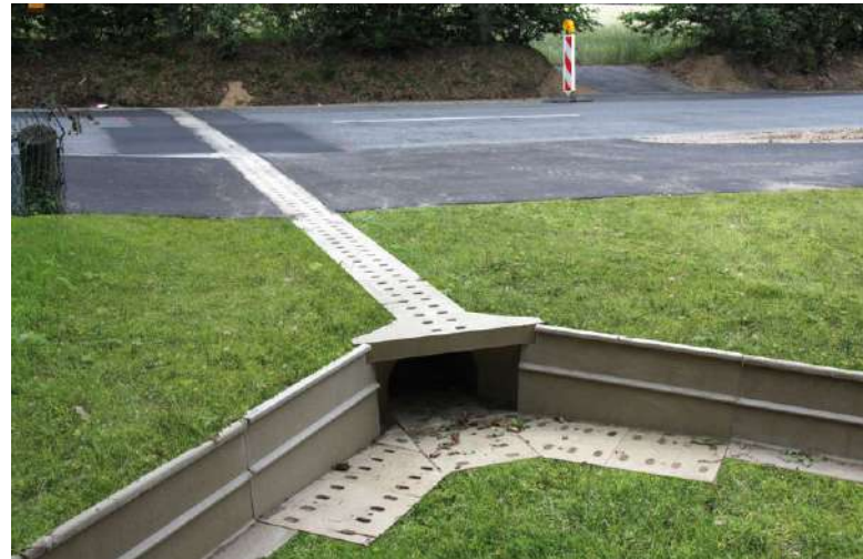
KT500 fauna tunnel
